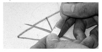
With the strip oriented so that the unexposed adhesive side extends over the gap, the exposed adhesive side is set down on one side of the tear with the leading edge of the polyester film as close to the edge of the tear as is comfortable. Apply brief pressure to establish the initial bond.
